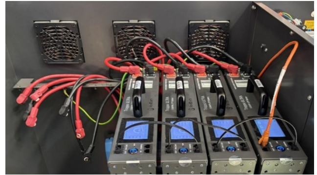
Connecting the DC power and comms cables (4 battery example)
